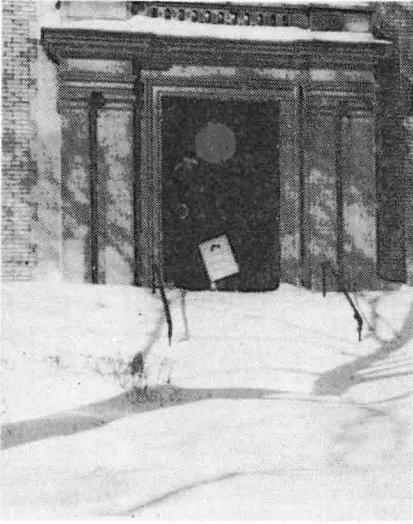
The front door of St. Matthew's Lutheran Church for the Deaf, Newark, N. J., on Sunday, Feb. 5, after a 22-inch snowfall. The sign on the door reads, "Use side door"
