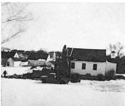
Silent Lutheran Church before the addition undertaken and completed during 1960
