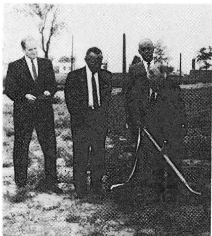
Mr. Walter Maack, president of Holy Cross Lutheran Church for the Deaf, St. Louis, Mo., breaks ground in a special service on Aug. 22 to announce the beginning of the building of their new chapel. Watching Mr. Maack are (from left to right) Mr. Rex Becker, architect; Mr. E. Mohme, Sr., chairman of the Friends of the Deaf; and Rev. John Ott, Vice-President of the Western District of our Lutheran Church. Rev. Floyd Possehl, present pastor of the St. Louis Field, is not pictured
